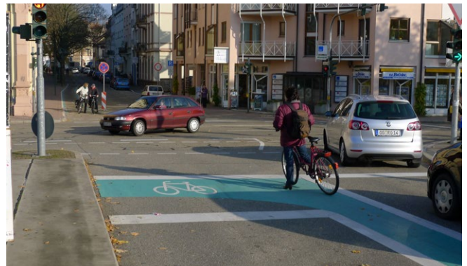
Bicycle box for safe turning left (Offenburg)
