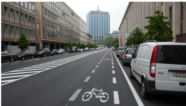
Brussels: Transformation of a four lane main street to a two lane street with cycle lane by new road markings
