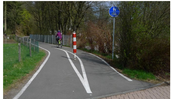
Visual contrast at bollard to prevent one-sided accidents (Cologne region)
