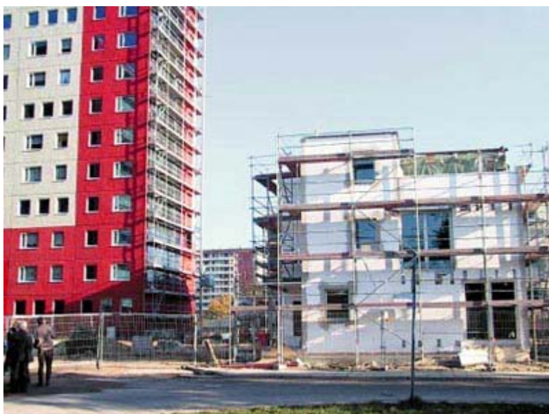
Redevelopment potential: Recycling of prefabricated panels to build suburban villas (Source: IRS, Erkner)
