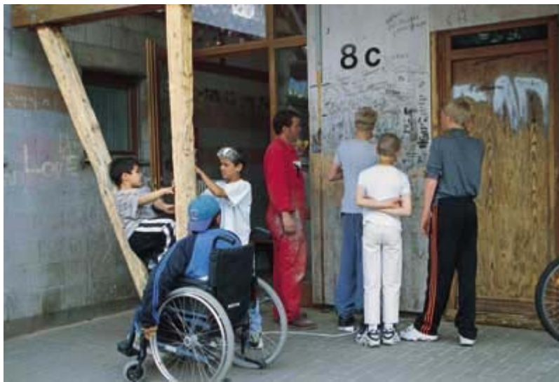
Remedial work on the children's house (Source: empirica, Berlin)
