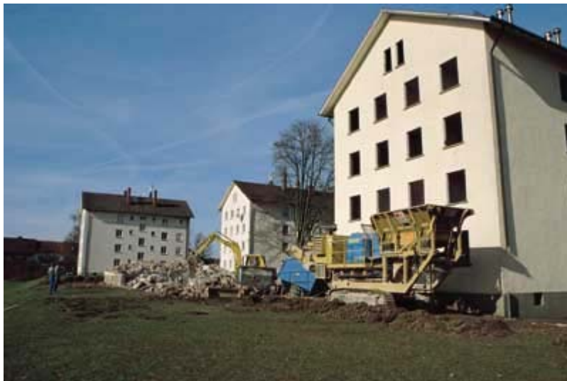
"Careful" demolition (Source: empirica, Berlin)
