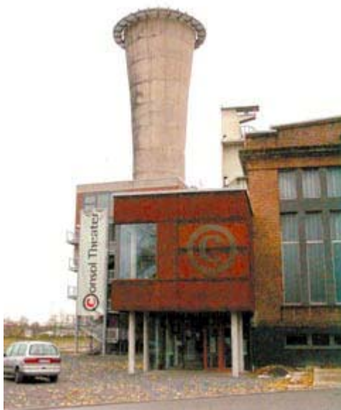
A ventilator machine building at the former Consol mine was converted by the "forum kunstverein" into a children's and youth theatre with restaurant and café. (Source: District Bureau Bismarck/Schalke-Nord)
